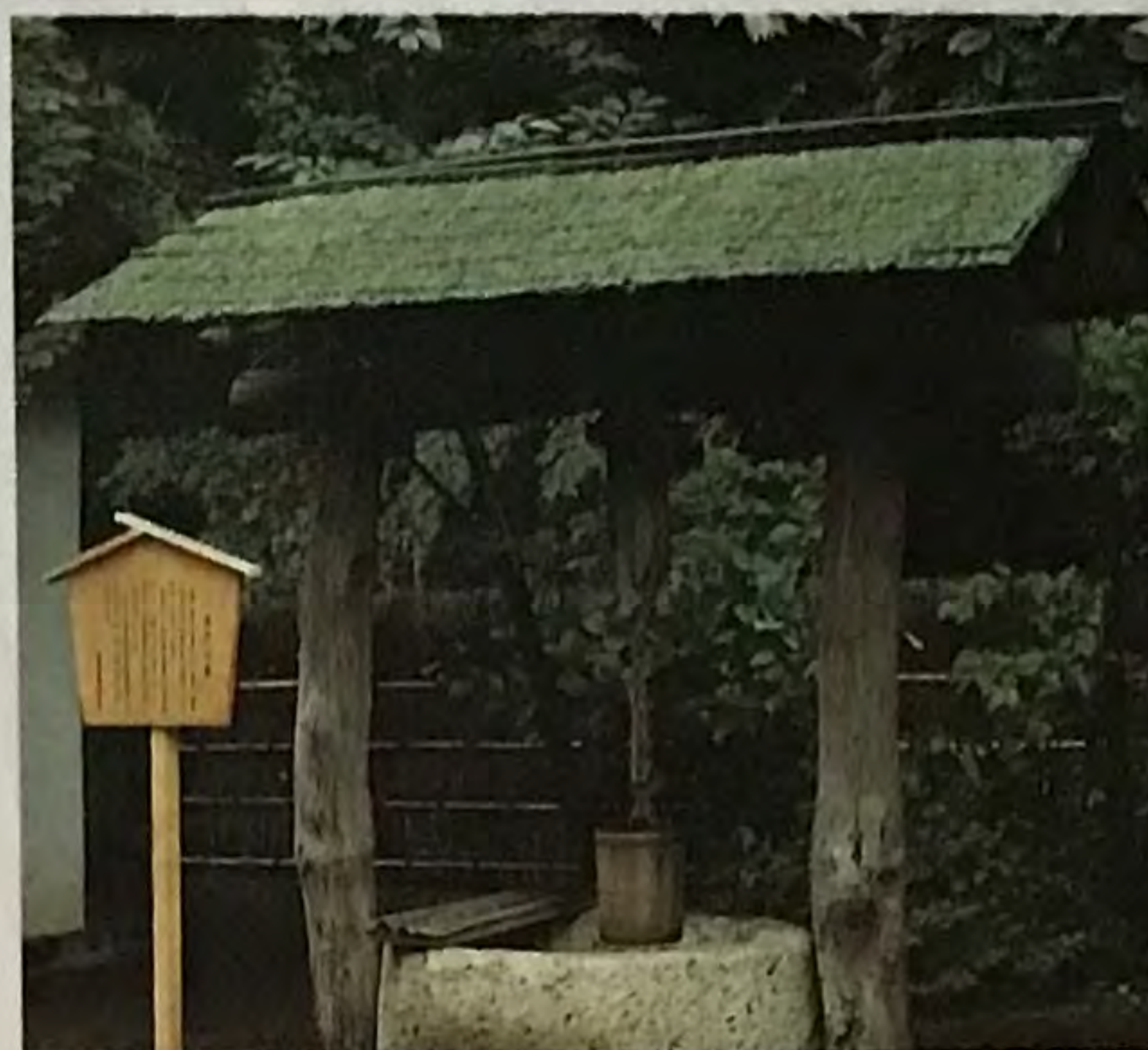
▲ The water piped from the underground water main was kept in a well like tank and drawn from there. Rich households built stones around the well as shown in the photo to keep sewage from flowing into it.
