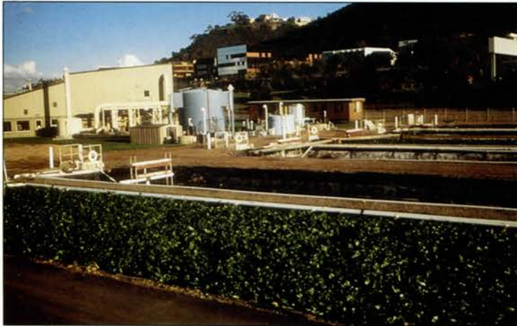
Aqua II Facility - Primary Treatment Building and Hyacinth Ponds
