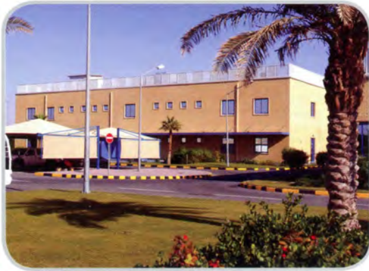
وٲٲٲٲ Administration Building
