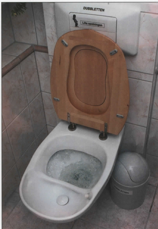
The two urine-separating toilets studied in this project and the project Recycling source separated human urine: on the left, the Dubbletten from BB Innovation & Co AB and, on the right, the DS toilet from Wost Man Ecology AB (previously WM-Ekologen AB).
