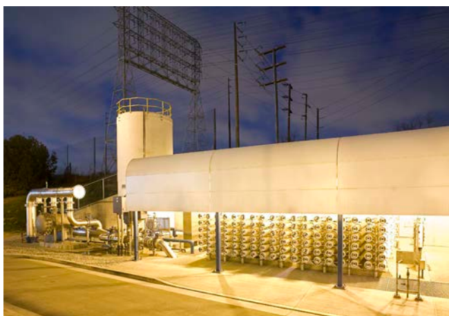
Figure 2 Reverse osmosis treatment at the ECLWRF
