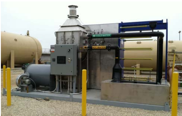
Figure 1 400 gpm Wastewater Pasteurization Demonstration System in Ventura California (Photo credit: Greg Ryan, Pasteurization Technology Group)
