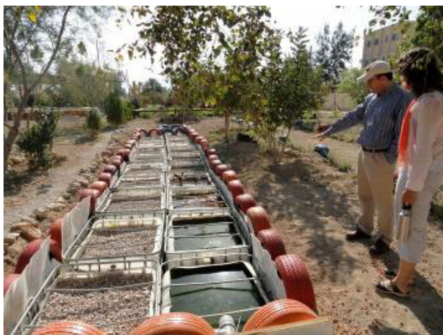
Figure 2 Graywater reuse system
