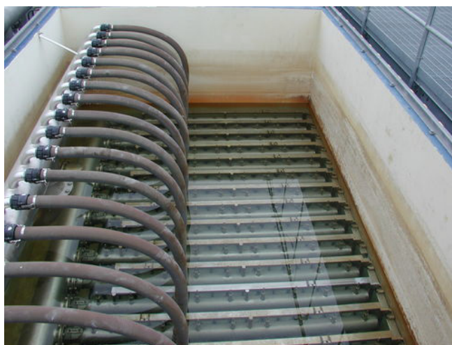
Figure 1 GWRS microfiltration system (Photo Credit: Gina DePinto)
