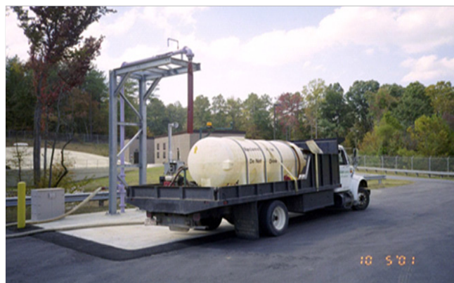
Figure 5-14 Cary, N.C., bulk fill station allows approved contractors, landscapers, and town staff to use reclaimed water
