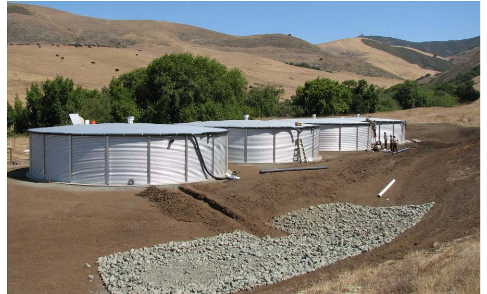
Rainwater catchment project near Pennington Creek, California, installed in partnership with the Morro Bay National Estuary Program, stores up to 296,000 gallons of rainwater for cattle troughs in the dry season.
