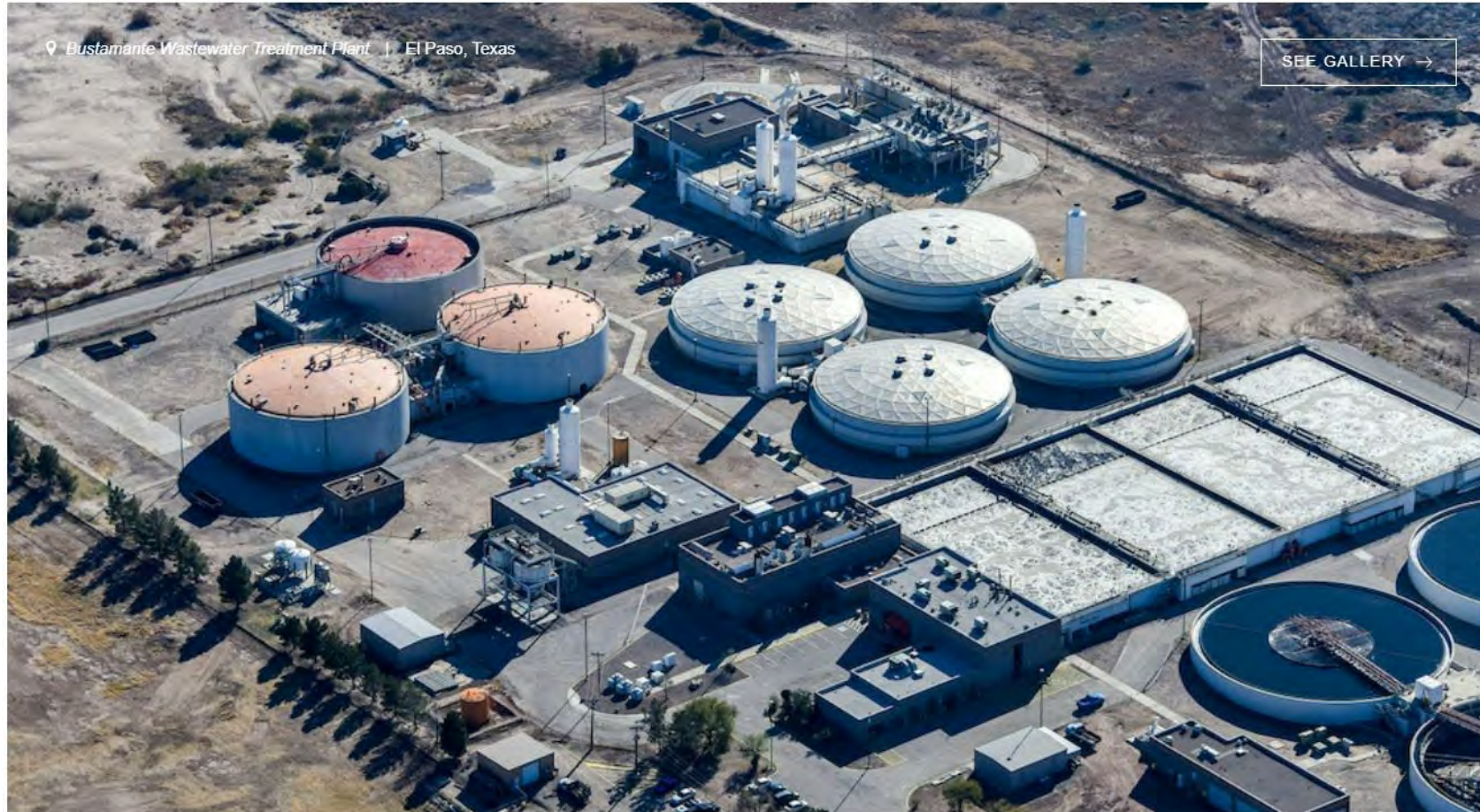
Bustamante Wastewater Treatment Plant secondary effluent Courtesy of Parkhill
