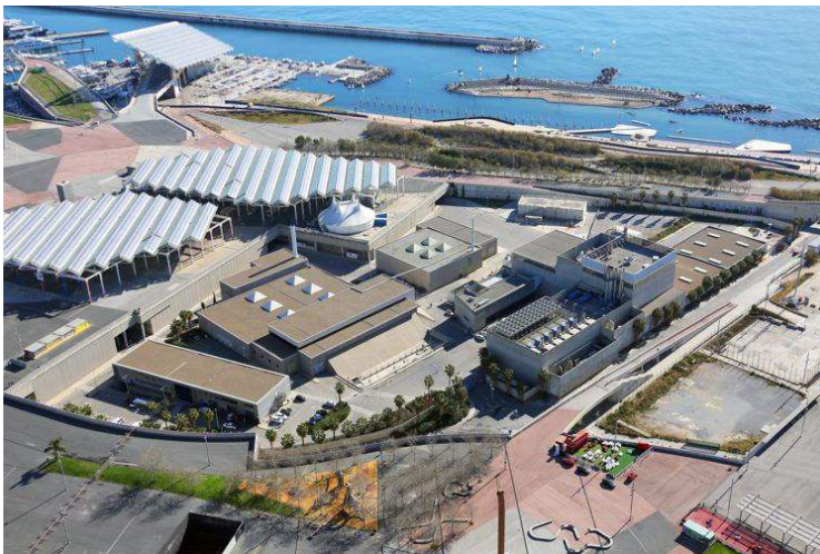
Besòs Wastewater Treatment Plant (Barcelona)
